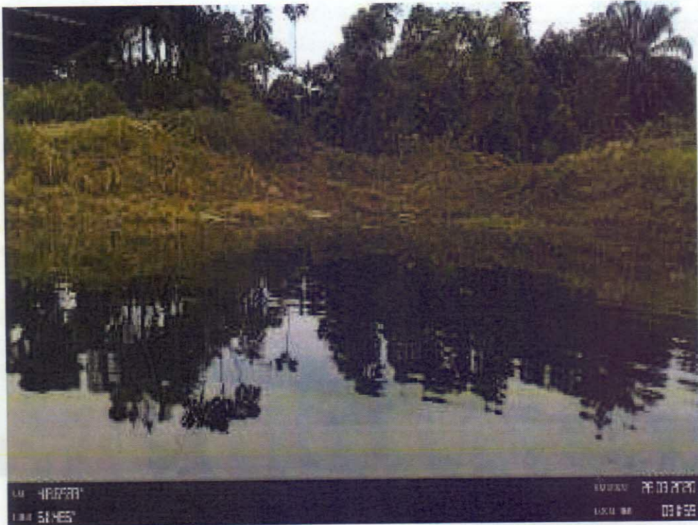
WITHERED VEGETATION AROUND THE SPILL POINT AREA
